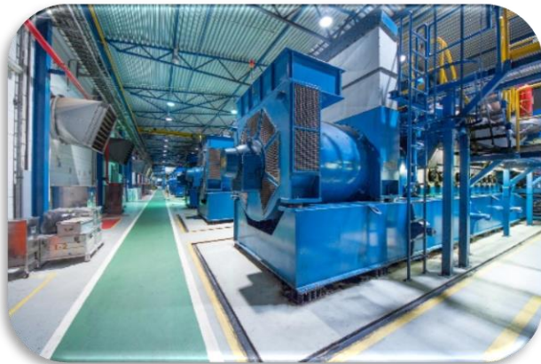
Figure 1. Engine generators at the power plant Tevisa located at Espírito Santo powered only by heavy fuel oil.
